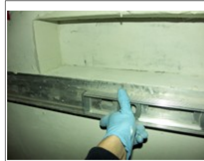
5: Using straightedge and level on corners
