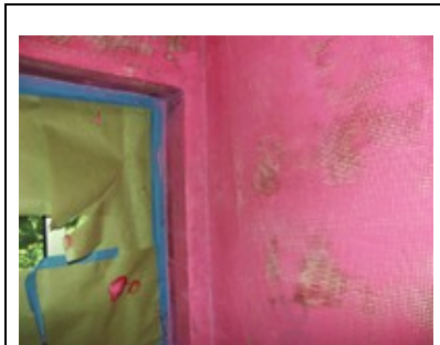
2: Fiberglass mesh embedded in Red Gard
