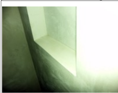
8: Second Base Coat Detail
