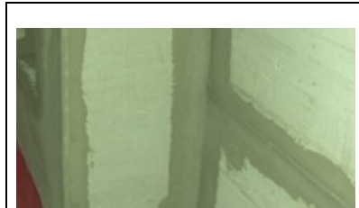
1: Embed 4" mesh with Milestone on the seams of the cement board
